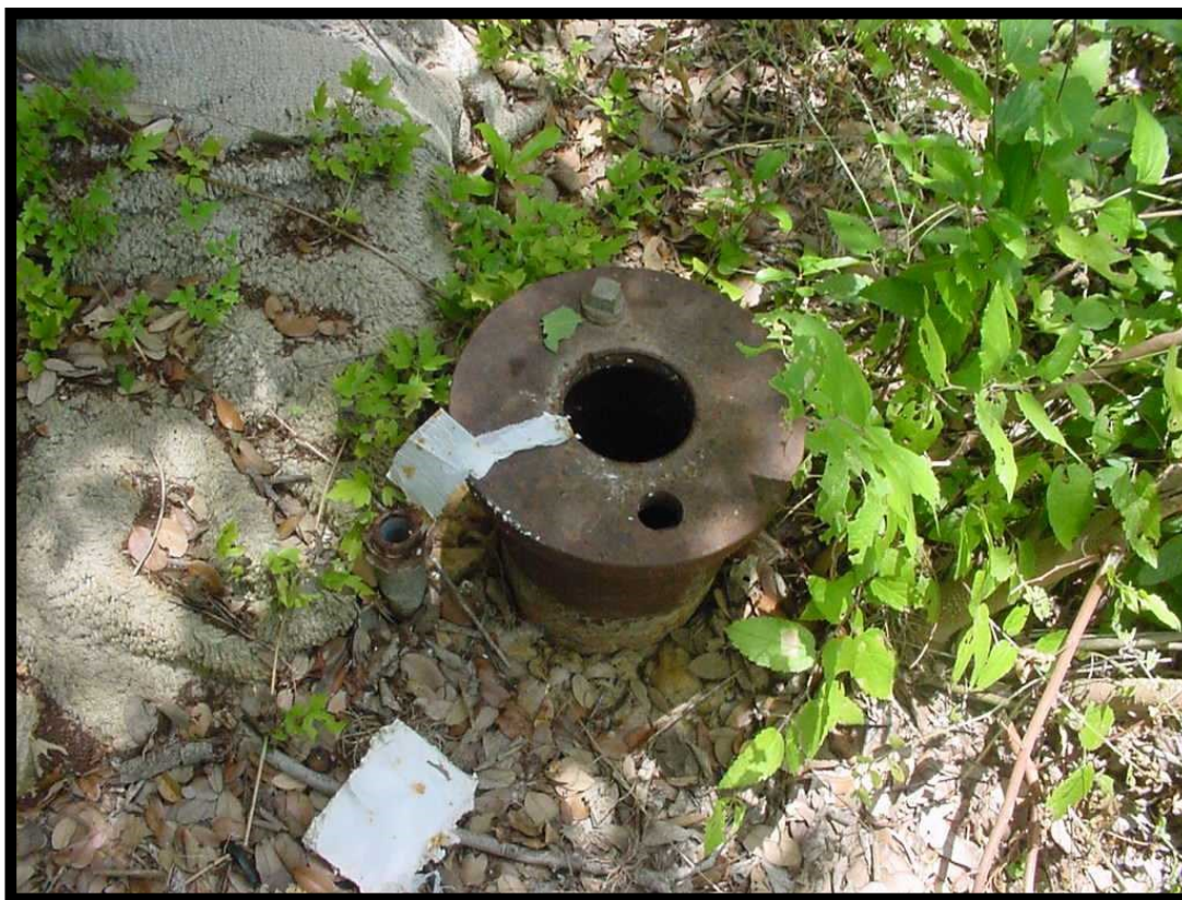
Figure 2. A unique way of utilizing an abandoned well (Courtesy of Geary Schindel of EAA). The white paper on and around the well is a toilet paper.
